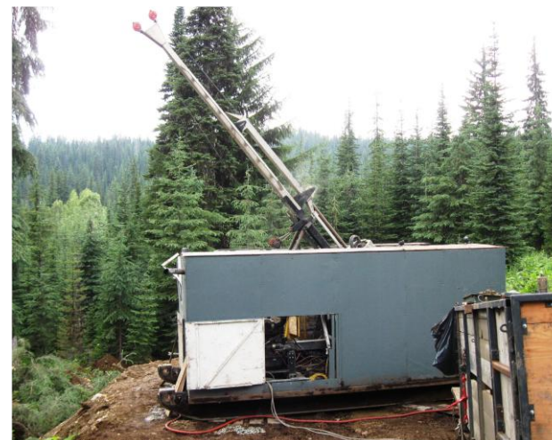
Drilling At Swift Katie
